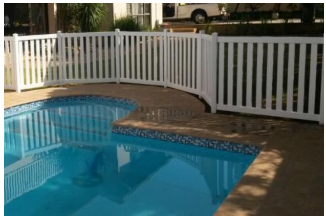
Pool Fencing and Pool Gates
